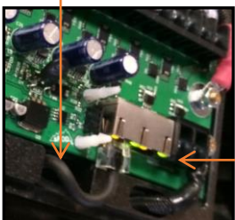
NOTE These lights are disabled and will not be on
